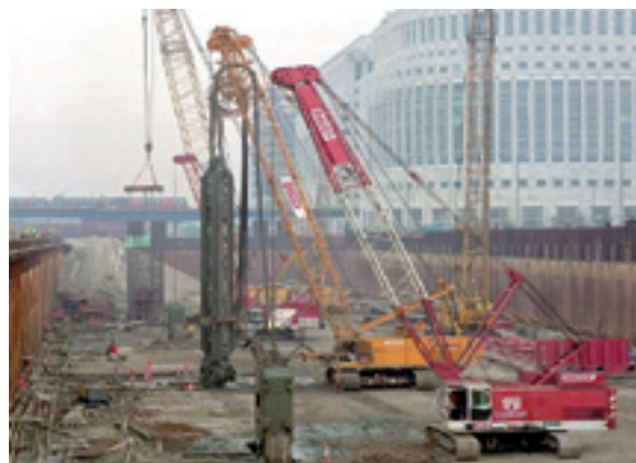
Slitsmursinstallation vid tunnelbanestationen Canary Warf i London Docklands.
